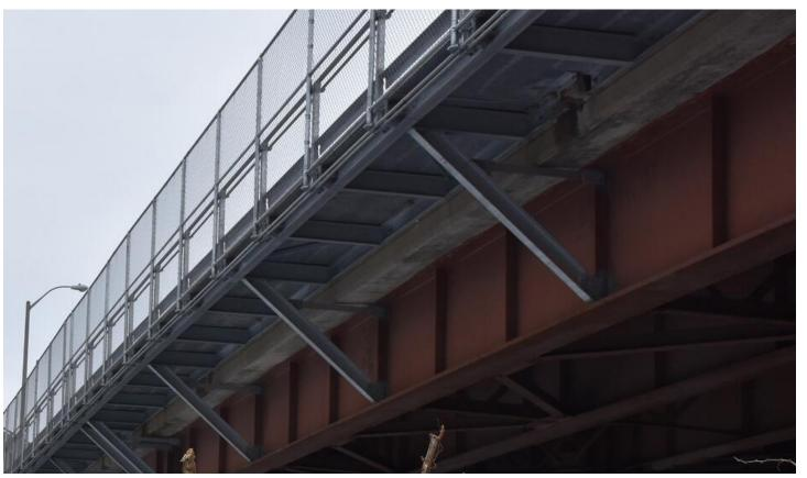
Example of a Cantilevered Sidewalk Bridge Addition
