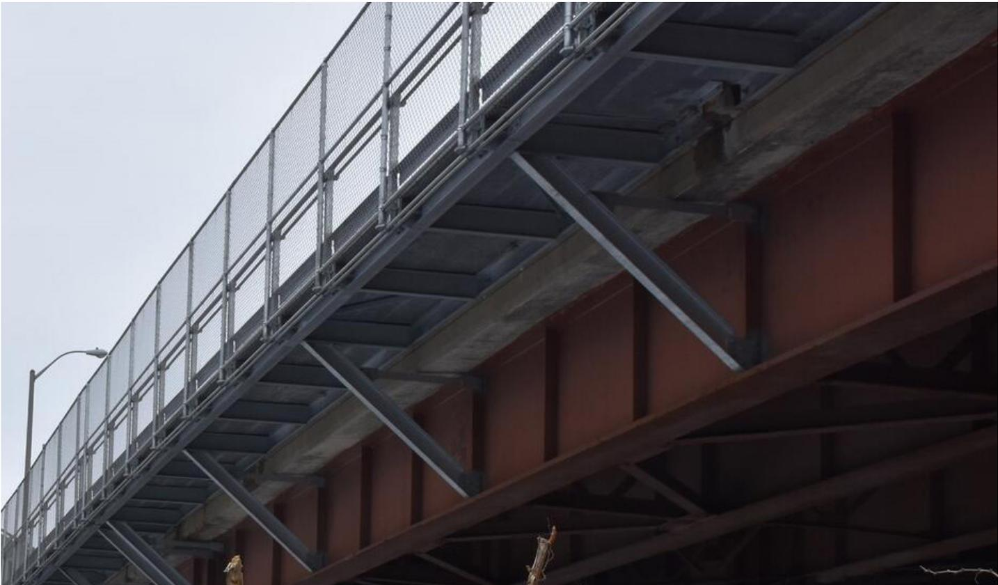
Example of a Cantilevered Sidewalk Bridge Addition
