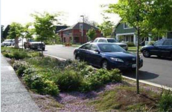
Bioswales are vegetated, mulched, or xeriscaped channels that provide treatment and retention as they move stormwater from one place to another. Vegetated swales slow, infiltrate, and filter stormwater flows. As linear features, they are particularly well suited to being placed along streets and parking lots.
