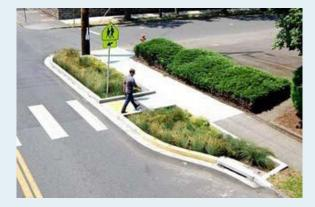
Green streets are created by integrating green infrastructure elements into their design to store, infiltrate, and evapotranspire stormwater. Permeable pavement, bioswales, planter boxes, and trees are among the elements that can be woven into street or alley design.
