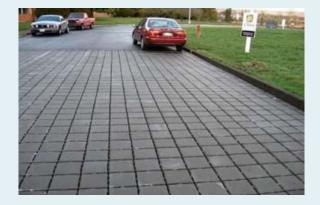
Permeable pavements infiltrate, treat, and/ or store rainwater where it falls. They can be made of pervious concrete, porous asphalt, or permeable interlocking pavers. This practice could be particularly cost effective where land values are high and flooding or icing is a problem.
