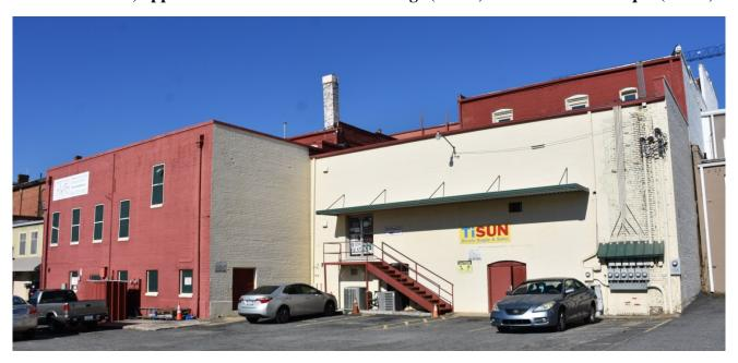
The north addition's six-to-one common-bond brick walls have been painted. The north and south elevations are blind. On the west elevation, painted plywood covers short square one-story window openings and second-story openings that contained one-over-one sash. All window openings have slightly projecting header-course sills. A single-leaf steel door is located at the first-story's center.
